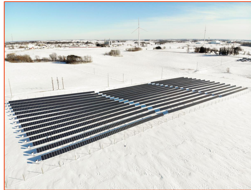
Endicott Community Solar Project, Cashton, WI
